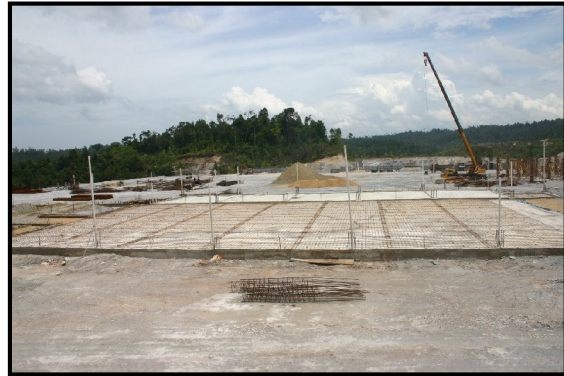
Administrative and Multi Purpose Hall as at 26 September 2006.
